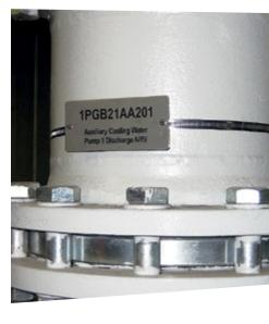
Our **identification plates** are produced in four materials to match the chemical and thermal environment they have to withstand:
