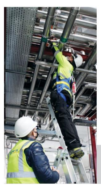
**ISO** 20560 is a new global standard ensuring uniformity in the marking of piping systems and tanks. This is the very first global standard which outlines a unified marking safety system for pipes and storage tanks. The uniformity of graphical symbols, coherent colour coding solutions and identical methods of information distribution are to ensure better recognition and quicker comprehension to enable an immediate identification of potential danger.
