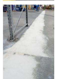
Elmetal removes all types of floor markings – lines, stripes, pedestrian crossings, arrows and other 5S shapes. The paint removal method is individually chosen to suit the particular type of surface.
