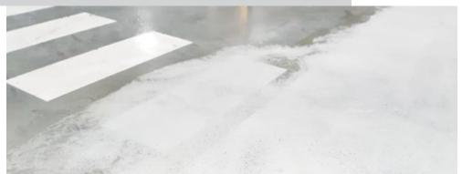
The removal of lines and floor markings is especially necessary after the reorganisation of traffic on circulation routes or after the expansion and modernisation of a production area. Sometimes, old floor markings are simply worn and illegible and therefore require repainting.
