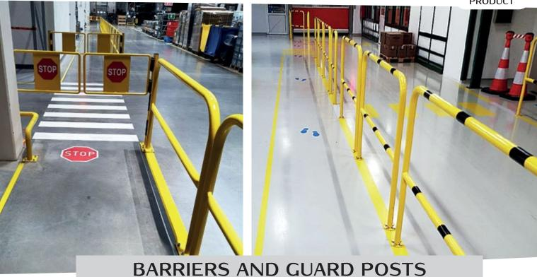
Industrial safety barriers are most often used in production plants or warehouses to separate pedestrian traffic zones from vehicular transport traffic areas. They can also cordon off and protect areas with equipment or machinery which is prone to damage.
